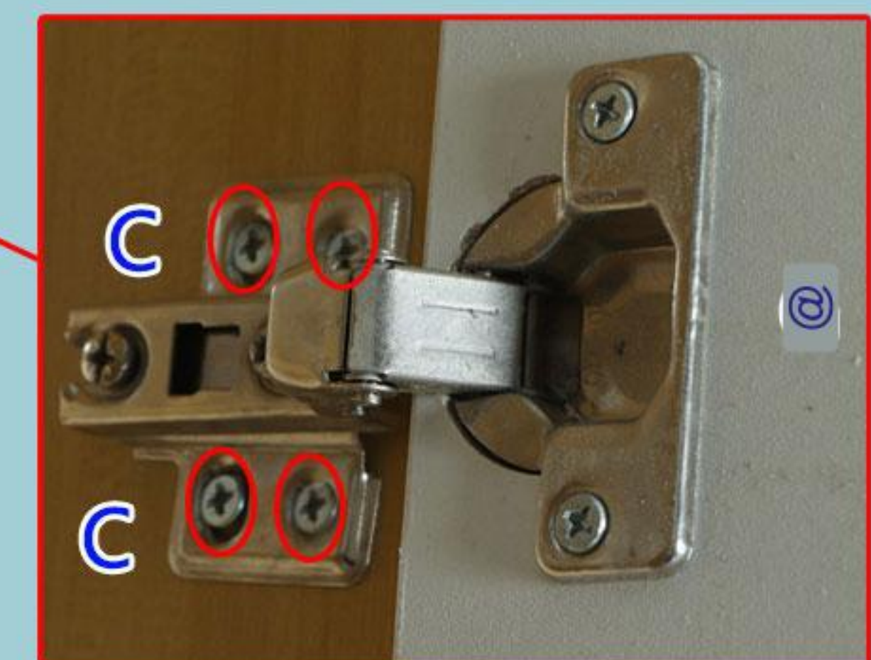
Screw in two screws first, and then screw in all the screws after the board is adjusted.
